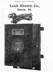
Trade Name—"Non Tune"; Type—Vibrator; operates from 110 volts, 25, 30 or 60 cycles, A.C.; Charging Rate— 2 amperes, 4 or 6 volts; Material of Case—Steel, enameled; Equipment— Ammeter; Dim.—5% x 6 x 9% inches.
