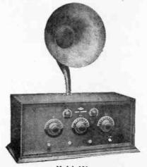
Model 100 Type-Neutrodyne; Tubes-5; Battery-"A" Storage; "B" 90 Volts; Built-in Loud Speaker; Price-\$100.00.
