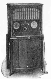
Model Radiola Super-VIII Model Radiola Super-Vill Antenna - Loop (self-contained); Tubes - 6 Battery--"A" Dry; "B" 90 Volts; "C" 4<sup>1</sup>/<sub>2</sub> Volts; Dim.-19 x 26<sup>1</sup>/<sub>2</sub> x 49; Wt.-98 lbs Controls-Tuning, 2; Station Selectors, 1 and 2; Price - With following equipment: Self-con-tained loud speaker and 6 UV-199 Radiotrons, K405 00 (Mat and arithet equipment) (Not sold without equipment.) \$425.00.
